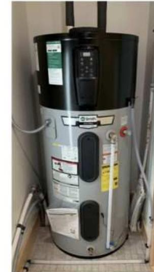
Figure 1. A heat pump water heater is installed in the interior closet of a multifamily dwelling unit. (Source: Larson Energy Research)
